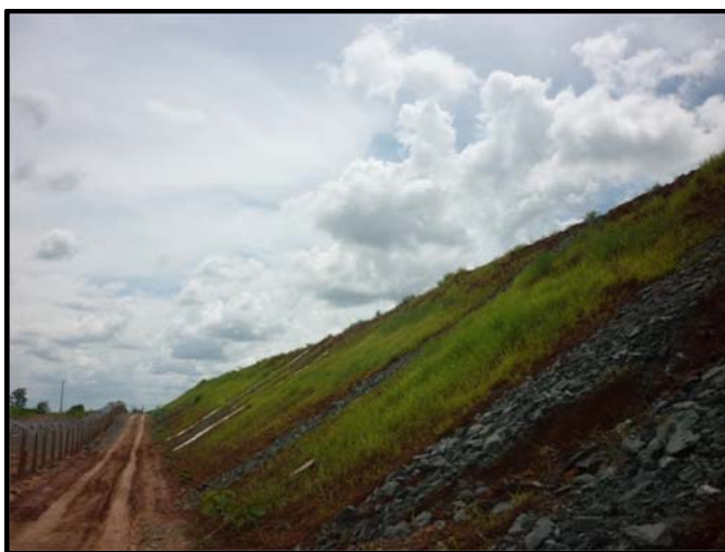
New Tailings Dam Construction
